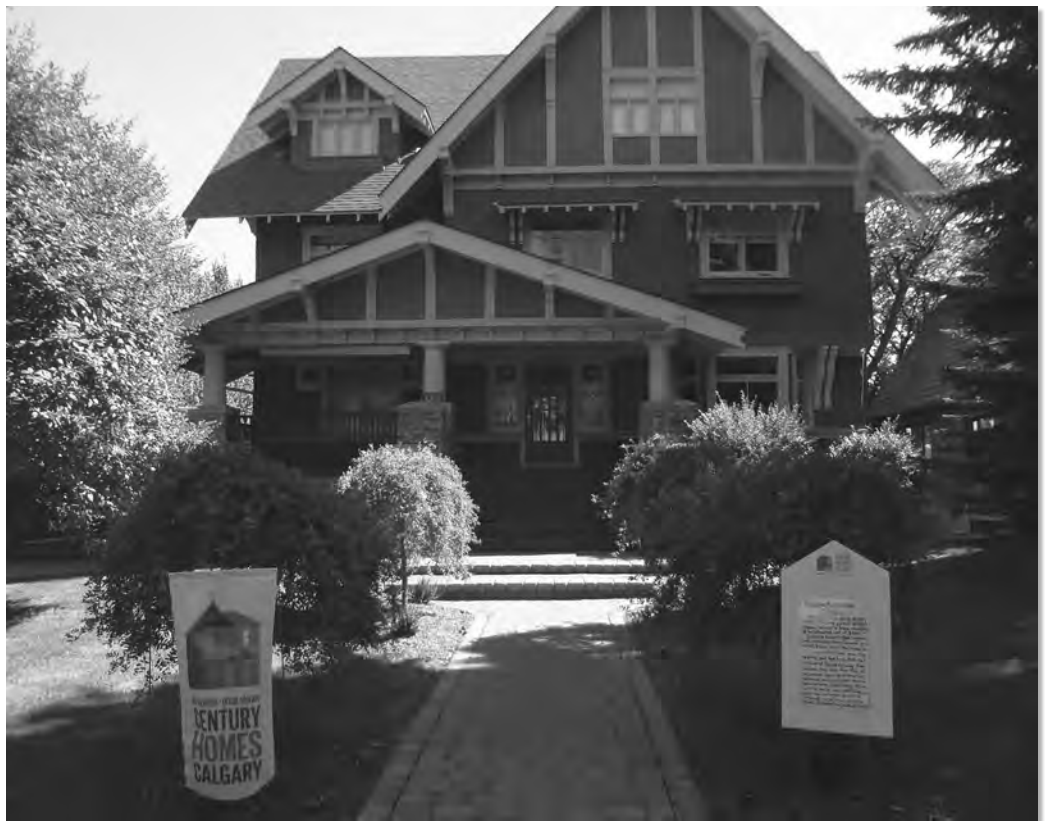
Fig. 3. Calgary's event celebrated the city's first building boom, when the railroad came to town. This bungalow was built in 1913. Courtesy of Cynthia Klaassen
