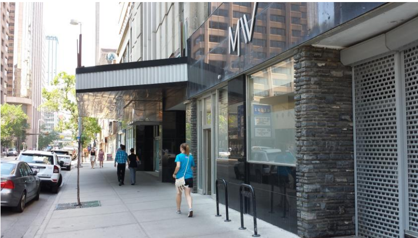
Marquee canopy today, ready for re-purposing
