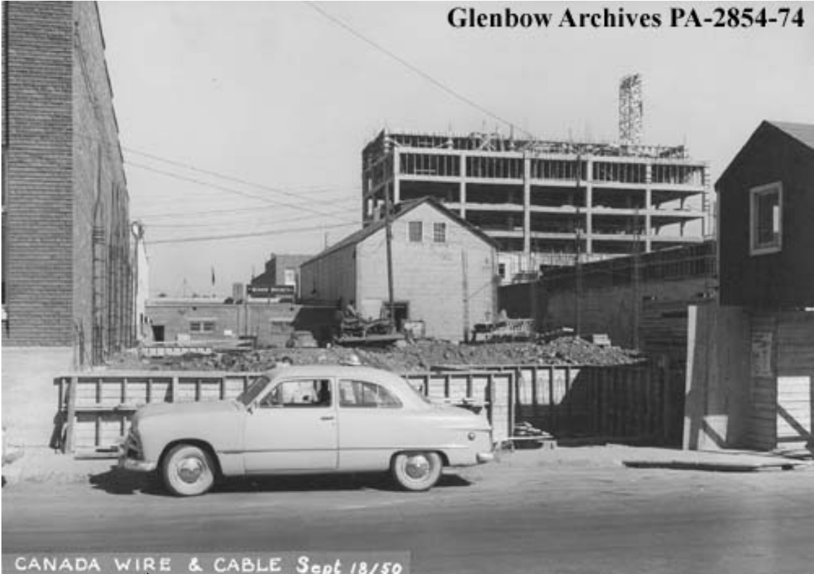
HP1 View from 9 th Avenue of Barron Building under construction 18 Sept 1950
