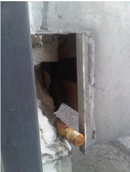
Photo 31 View of concrete & reinforcing bar at pilaster base
