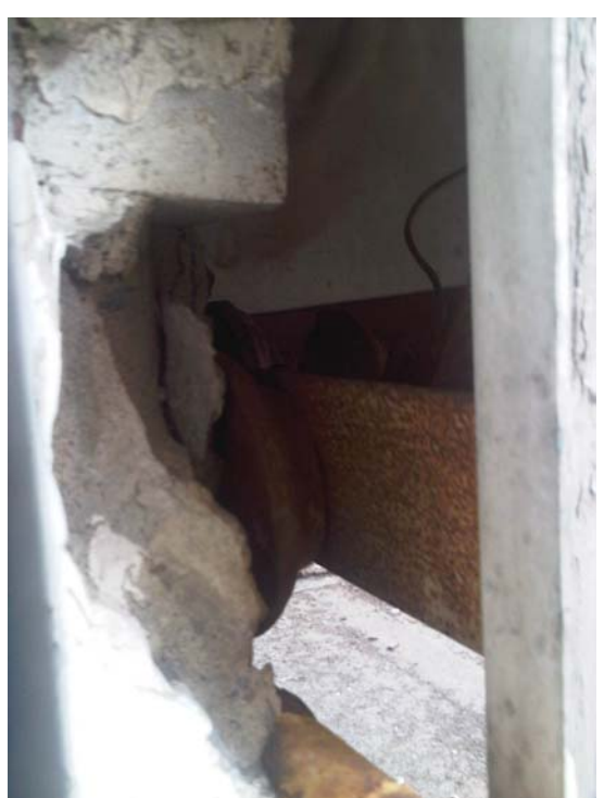
Photo 32 Detail view of steel connectors at pilaster base
