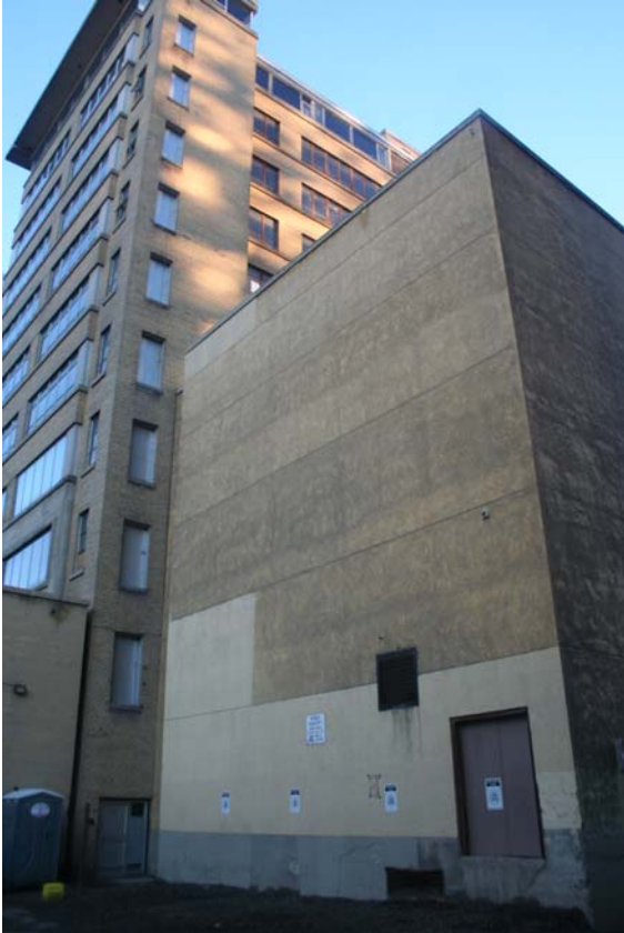
Photo 15 View of east façade of theatre looking SW
