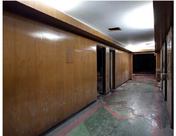
Photo 72 View of typical elevator lobby w/ office doors visible on left across from elevator doors on right
