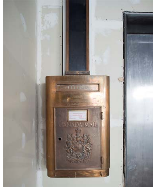
Photo 66 Detail view of mail box & chute in main floor elevator lobby
