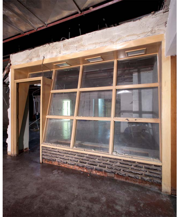
Photo 76 View of basement office of Jack Cawston
