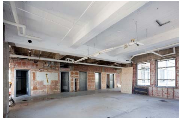
Photo 100 View from typical projection looking NE back at elevator lobby
