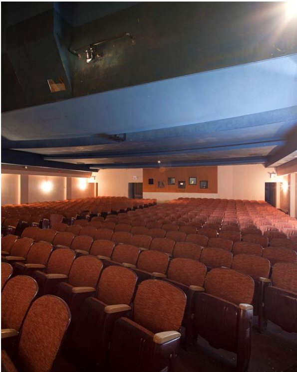
Photo 53 View across theatre seating to rear wall; front edge of balcony visible above
