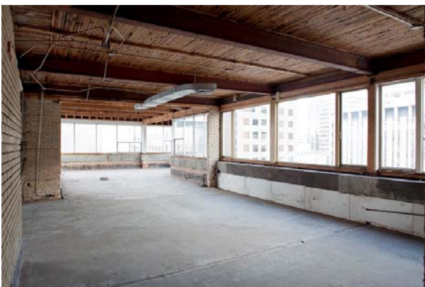
Photo 92 View of penthouse suite looking west; roof structure is wood & timber
