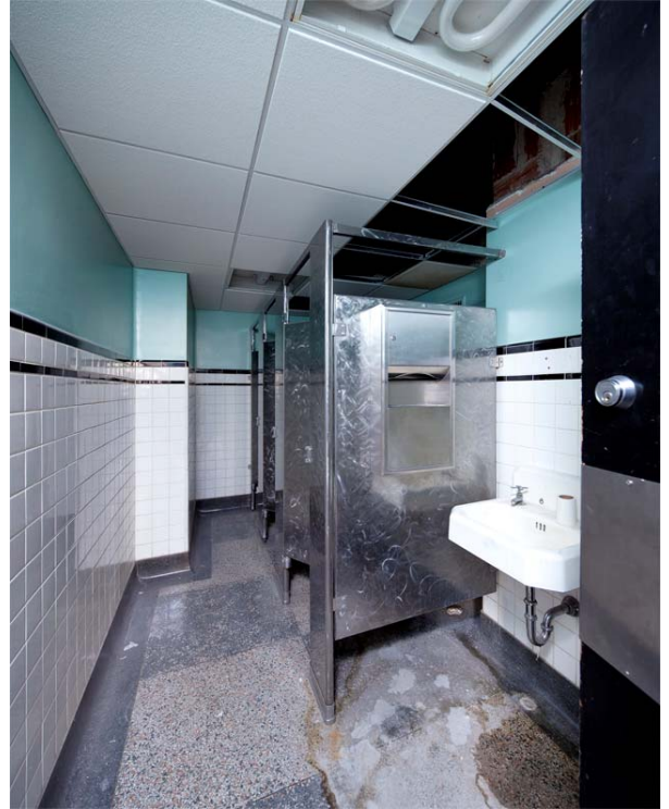
Photo 108 View of women's washroom in office tower
