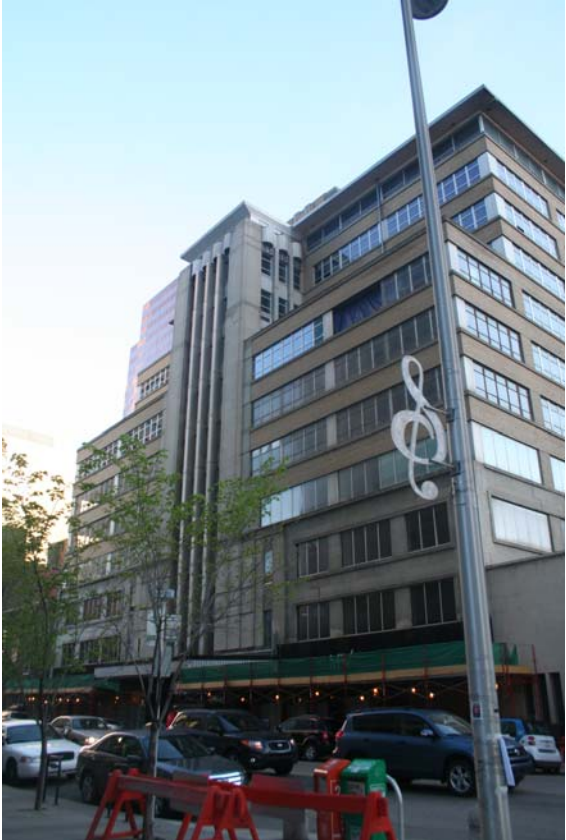
Photo 2 View of front façade looking NW
