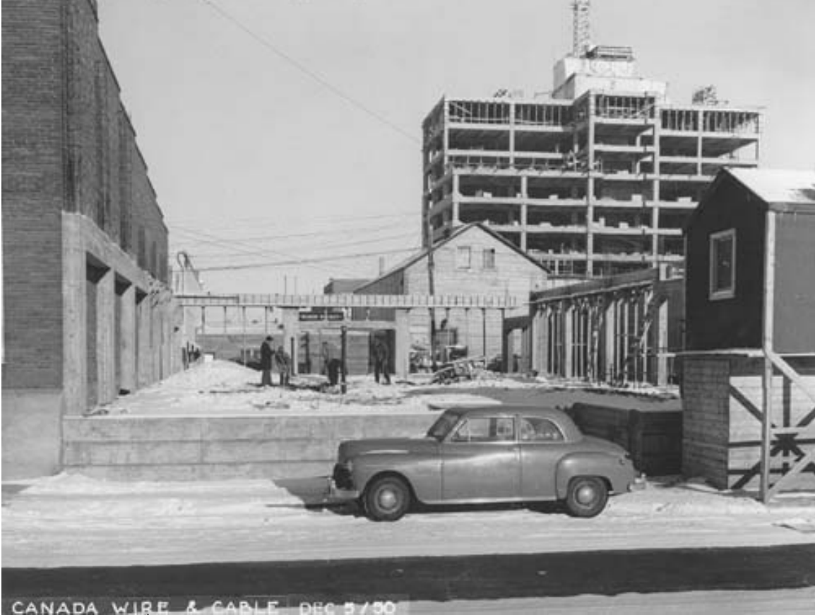
HP3 View from 9 th Avenue of Barron Building under construction ca. late 1950/early 1951
