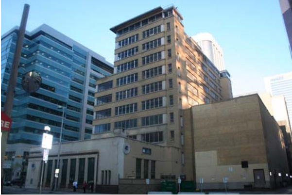
Photo 5 View of east & rear façades & theatre looking SW
