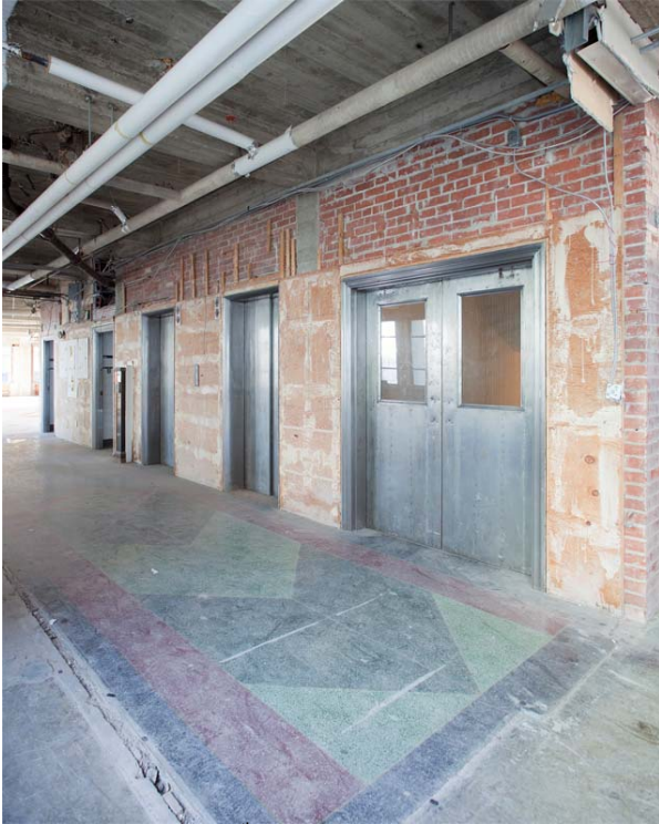
Photo 98 View of 10 th floor elevator lobby; demising partitions have been removed
