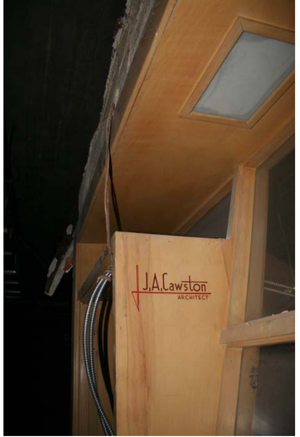
Photo 80 Detail view of entry to Jack Cawston's office
