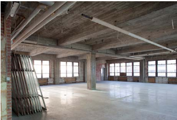
Photo 101 View looking NE toward exit door from elevator lobby area on 8 th to 10 th floors, typical
