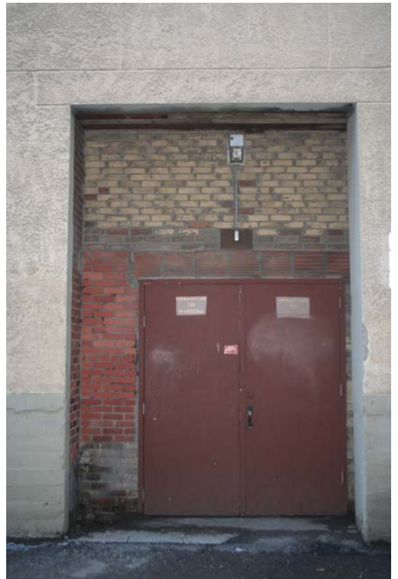
Photo 18 View of NW exit from office tower & theatre
