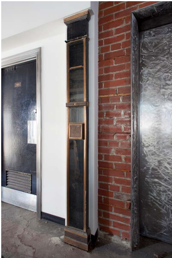
Photo 109 View of washroom door, mail chute, & elevator door typical for 4 th to 10 th floors
