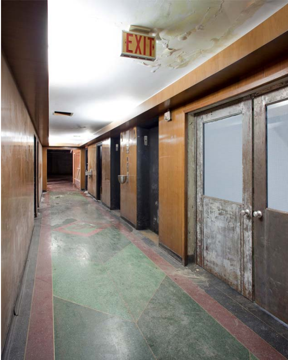
Photo 71 View of typical elevator lobby w/ exit doors at right, then 2 elevator doors, then 2 washroom doors
