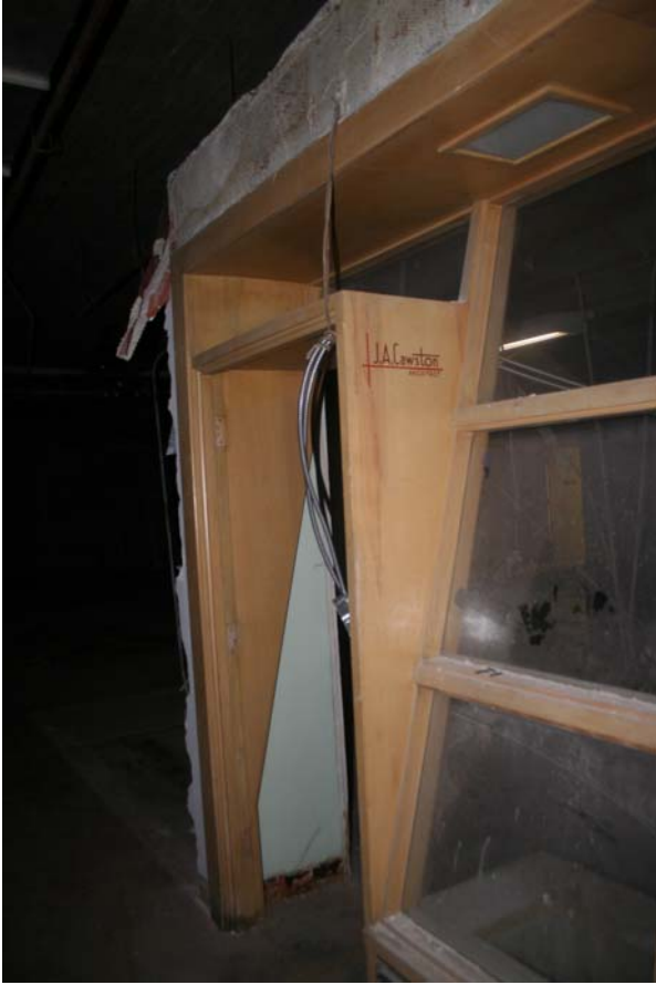
Photo 79 View of entry to Jack Cawston's office
