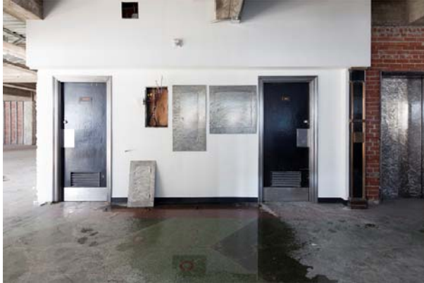
Photo 107 View looking toward washroom doors
