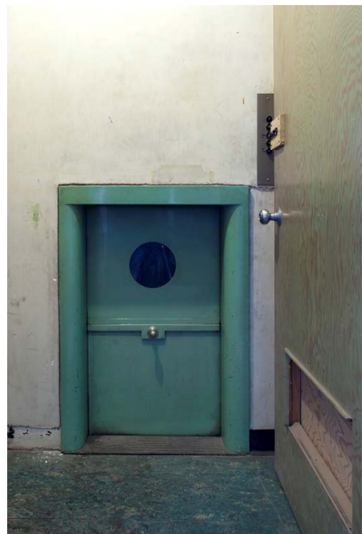
Photo 62 View of dumbwaiter beside projection booth
