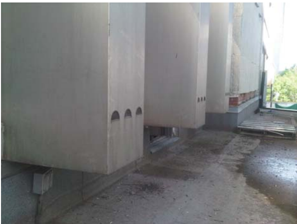
Photo 29 View of base of metal pilasters just above marquee
