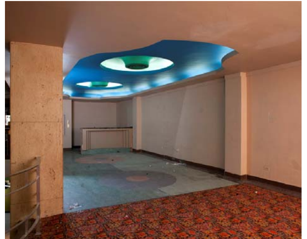
Photo 50 View of ceiling detail on west side of mezzanine level
