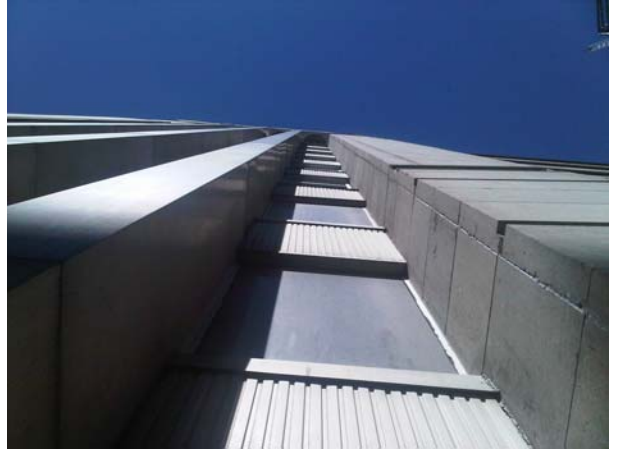
Photo 28 View w/ metal & limestone pilaster at right
