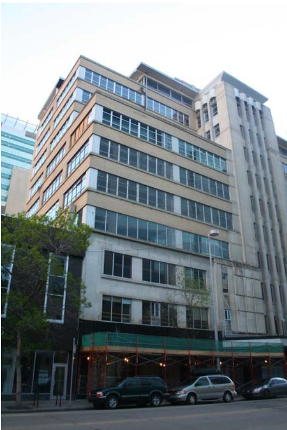
Photo 3 View of front façade looking NE across 8 th Avenue
