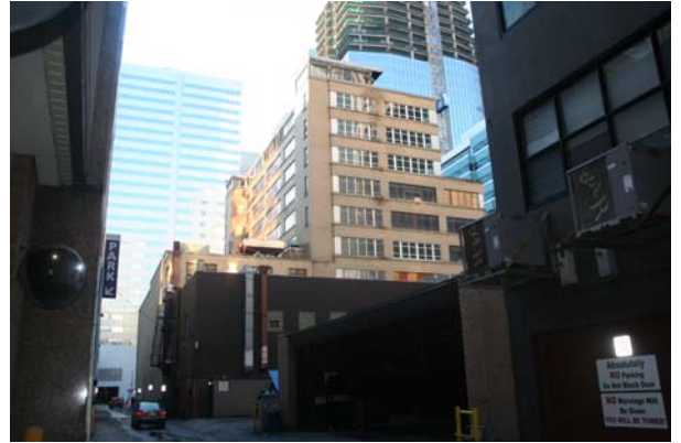
Photo 6 View of west & rear façades looking SE
