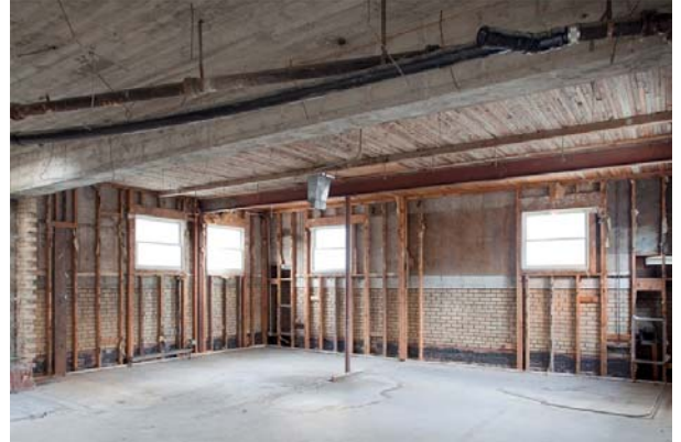
Photo 89 View of partially demolished penthouse suite
