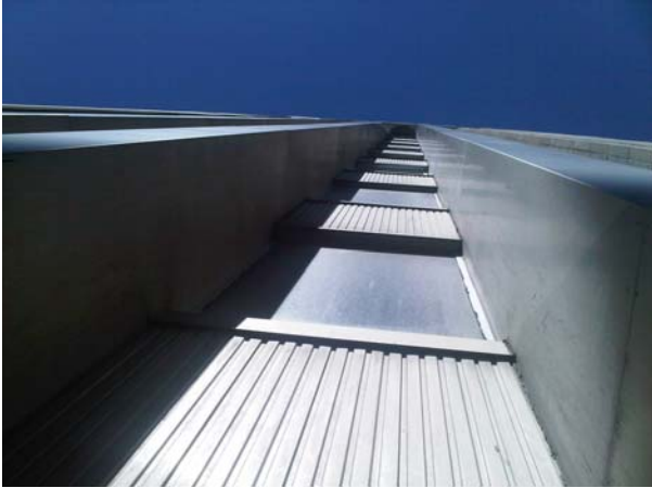
Photo 27 View up frontispiece w/ metal pilasters each side
