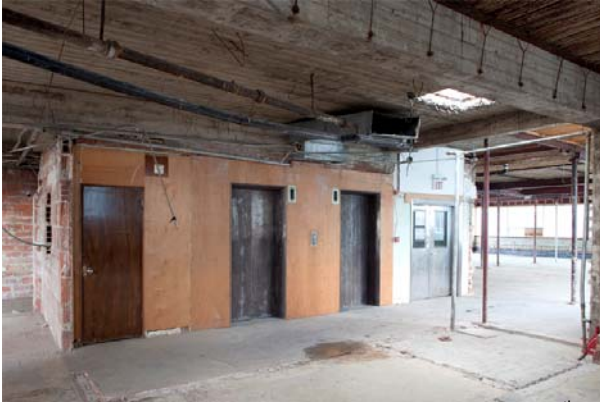
Photo 88 View of partially demolished penthouse (11 th floor) elevator lobby
