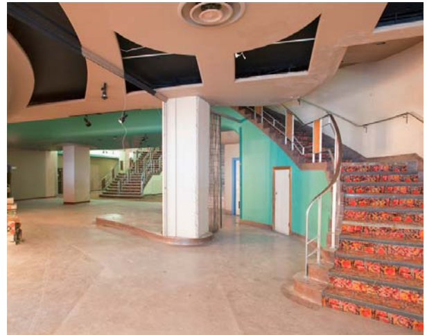
Photo 40 View of curved stair at right and toward grand stair up to mezzanine
