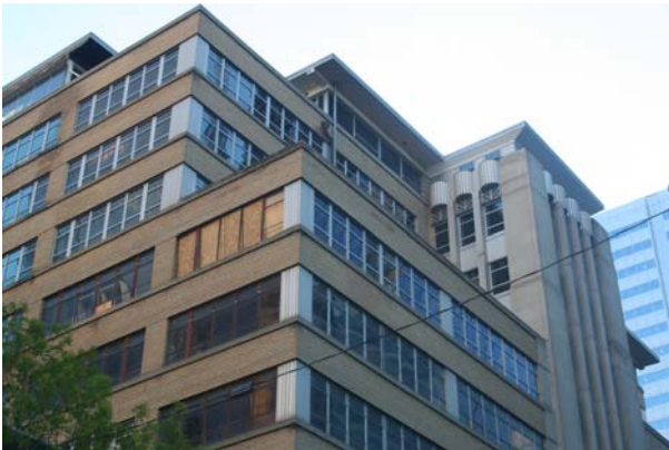
Photo 11 View of step back in upper storeys looking NE
