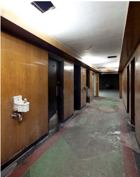
Photo 73 View of typical elevator lobby floors 2 to 10; walls and lighting cove constructed in hardwood veneer panels; multi-coloured terrazzo flooring w/ brass inlay
